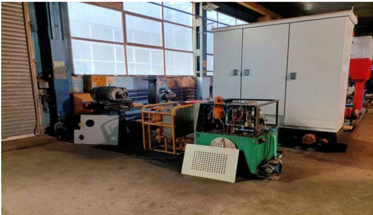
Fig 1- Standuri testare Instalatie de cimentare in zona dulapuri electrice
