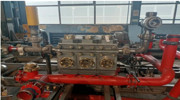
Fig. 3 Triplex pump with plunger
